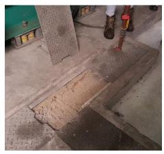
Sand filled trench containing fuel pipes (outside the fuel tank chamber)
