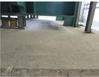
**BH8 View 1** - concrete floor condition underneath emergency generator
